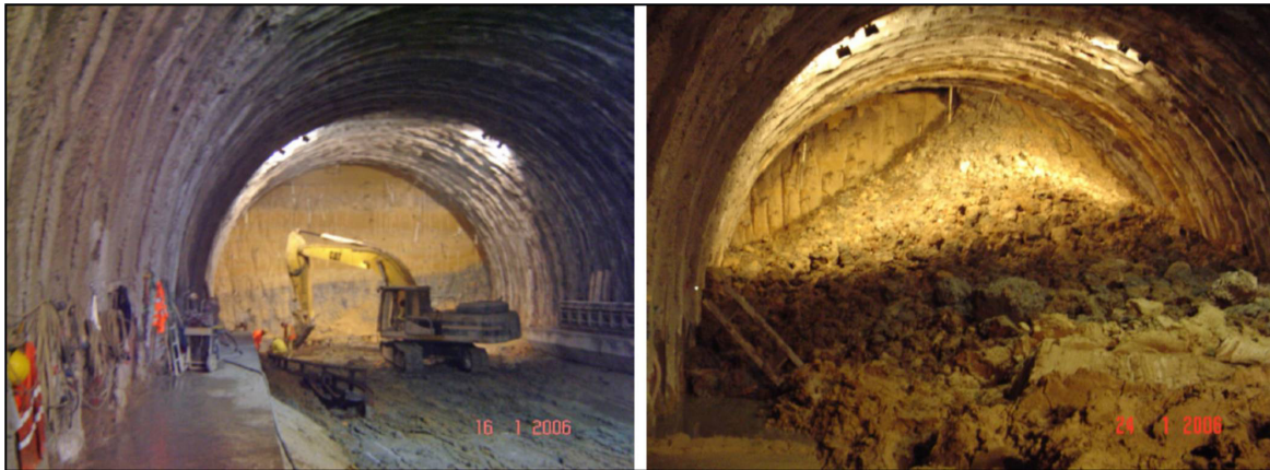
Figura 1: Fronte di scavo prima (a sinistra) e dopo (a destra) del verificarsi del fornello. Figure 1: Excavation forehead before (left) and after (right) the saturated inflow occurring.
