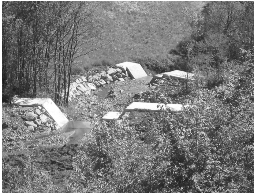
Fig. 5 Particolari briglie in gabbioni con gaveta Details about gabions's braces with concrete reinforcement
