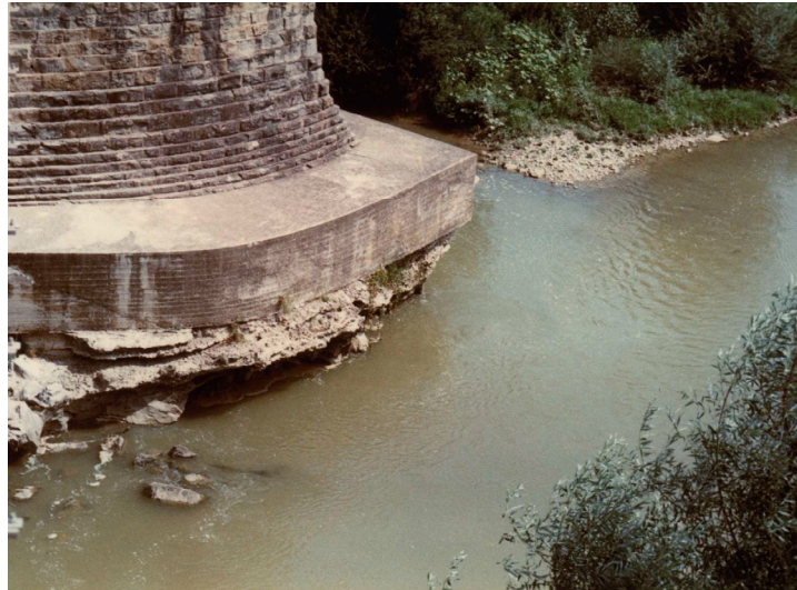
Fig. 5 – The lowering of the riverbed of the Arno River is creating serious problems for the stability of engineering works. In this picture the Terranuova Bracciolini Bridge, in Upper Valdarno, shows the precarious state of its foundations, in spite of the consolidation works carried out in the sixties (from CENCETTI et al., 1994).
