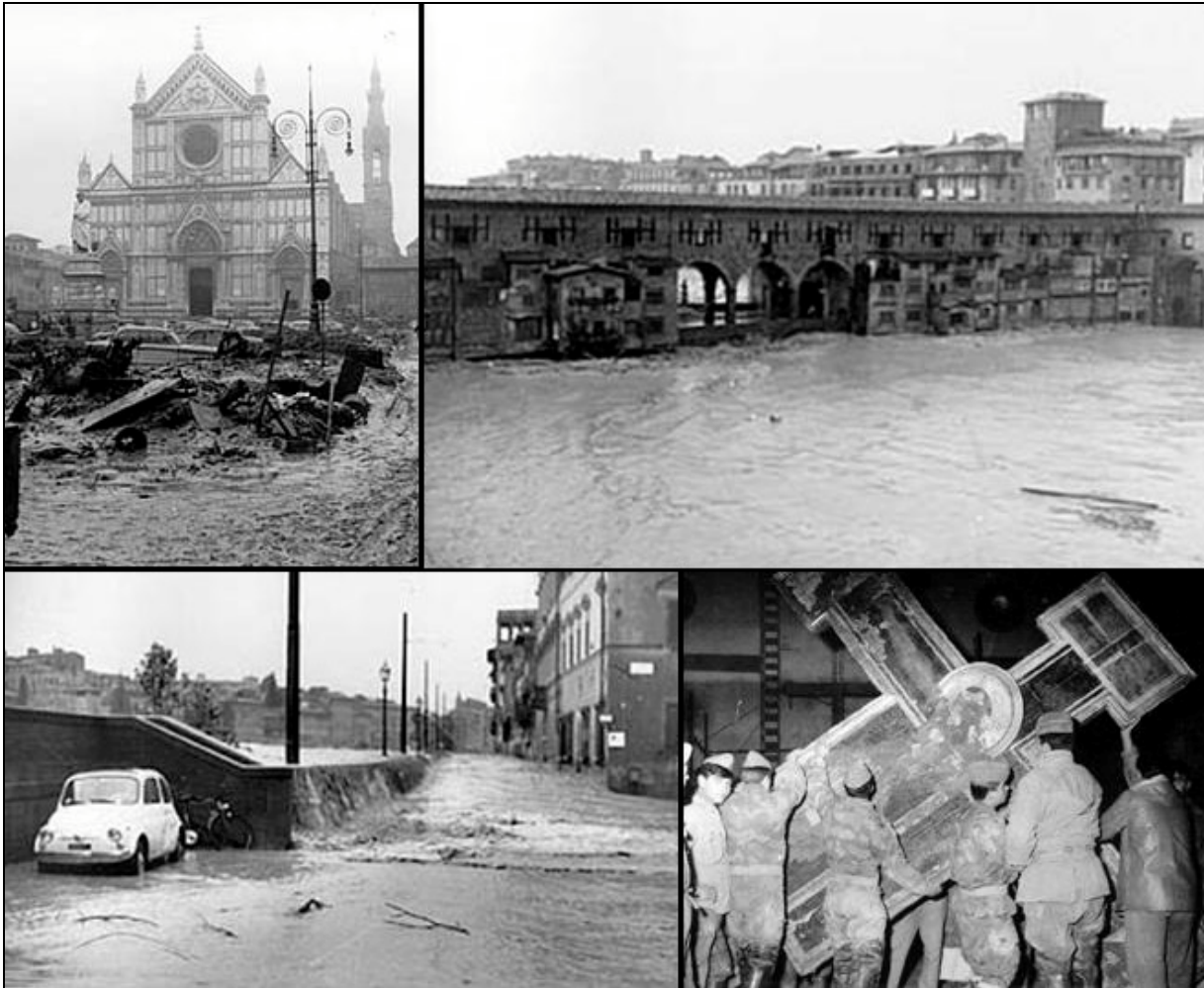
Fig.10. Pictures of the 1966 flood in the city of Firenze. Top left: flood effects in Santa Croce; Top right: the flood in Ponte Vecchio; Bottom left: overtopping of the banks in the city; Bottom right: the Cimabue crucifix seriously damaged by the flood in Santa Croce.
