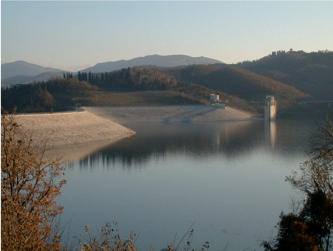
Fig.12 - The Bilancino earthfill dam impounding a reservoir of 17 \cdot 10^6 \text{ m}^3 in the upper Sieve basin.
