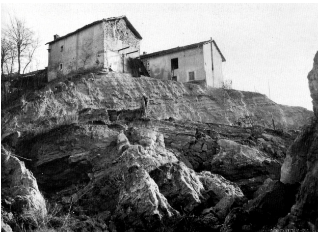
Figure 4 – Cigliè (Cuneo Province). Rock-block slide of January 1963: 10 buildings damaged and 17 others evacuated.
