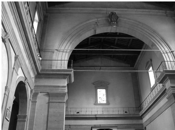
FIG. 3 – The interior of San Salvatore al Monte: on the arch some old restored cracks are evident.
