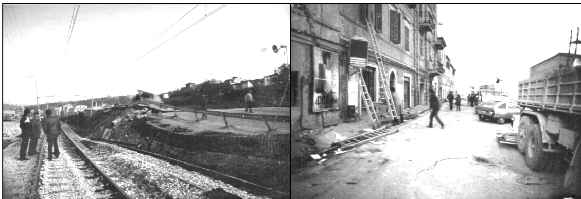
Fig. 1. Railway (a) and Flaminia Road (b) interrupted by the landslide.
