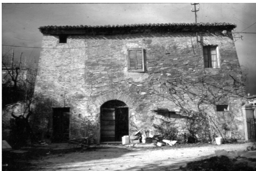
Fig. 7. The old postal-house sited on the T 2 trench. The house has undergone rotation, as can be recognized from the ancient repairs.
